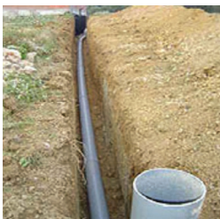
Canadian well installation
