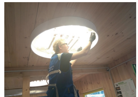
A photo that shows a student mounting DALI based LED illumination.
